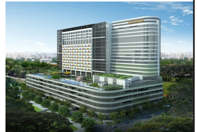
Figure 14. Connexion Integrated Health Center, Medical Hotel, Singapore
