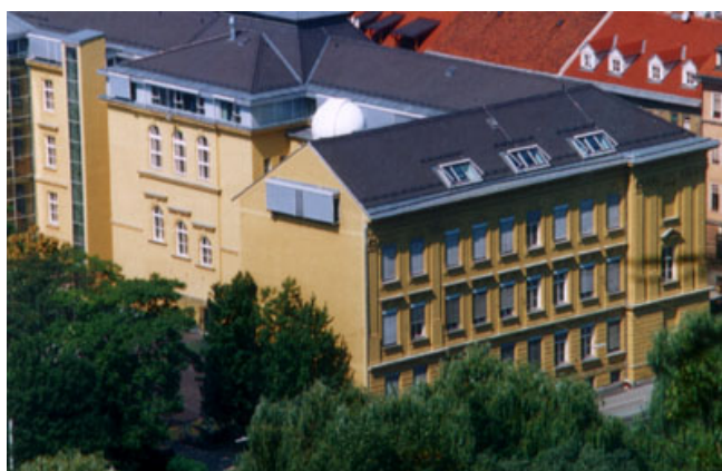
Figure 2.5: Picture of school building BRG Kepler 8
