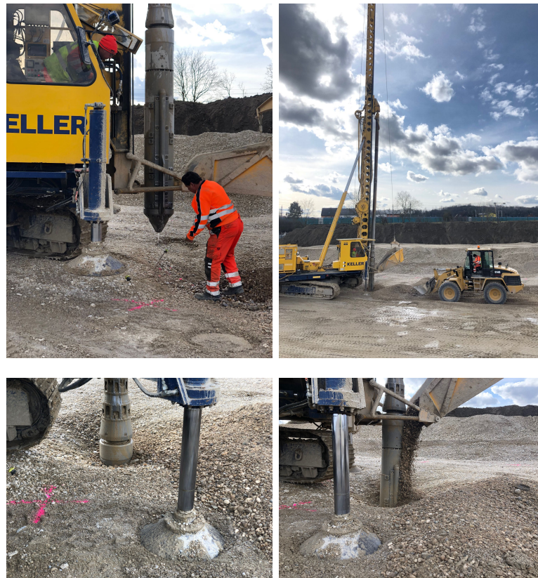
Figure 2.4: Procedure vibroflotation method - photographs
