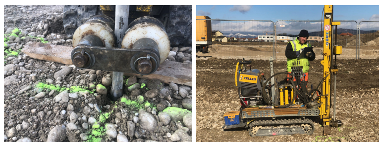
Figure 3.25: Dynamic probing heavy - test
