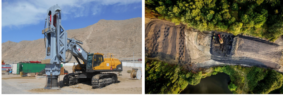
Figure 2.7: Impulse compaction method according to [12]
