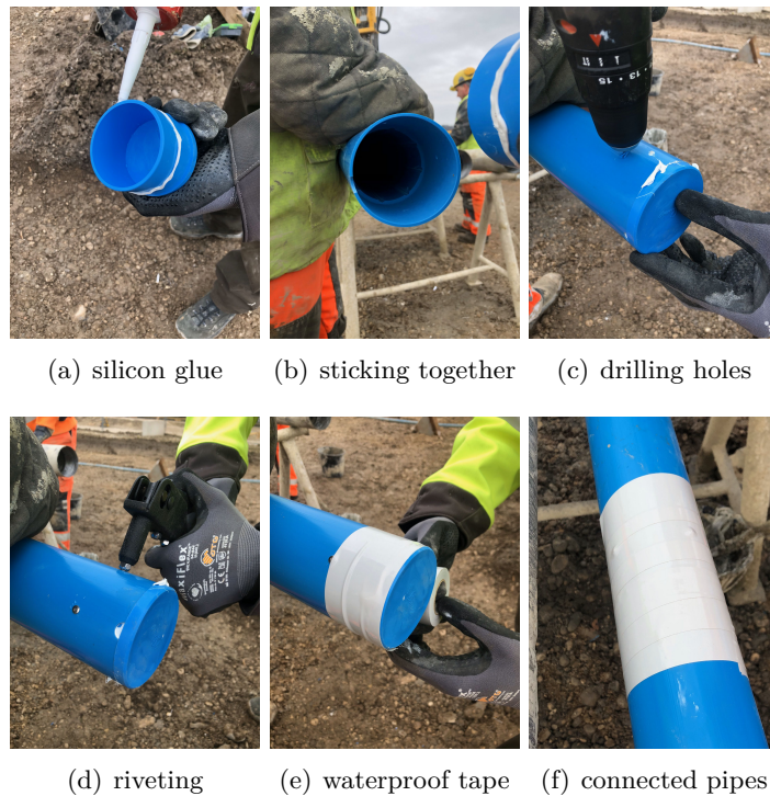
Figure 3.17: Connection of the inclinometer pipes
