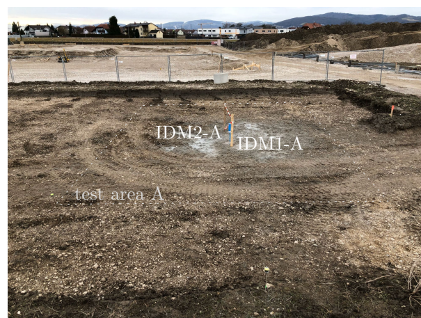
Figure 3.2: Test area A immediately after the installation of the inclinometer pipes
