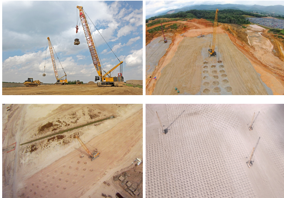
Figure 2.6: Dynamic compaction method according to [12]
