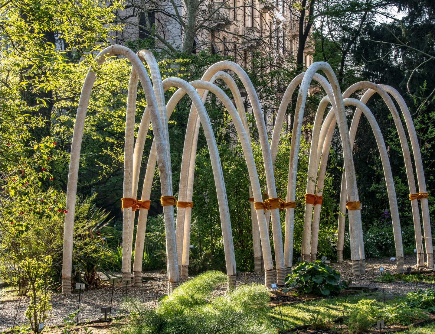
Fig. 35: Arch assembly - The Circular Garden
