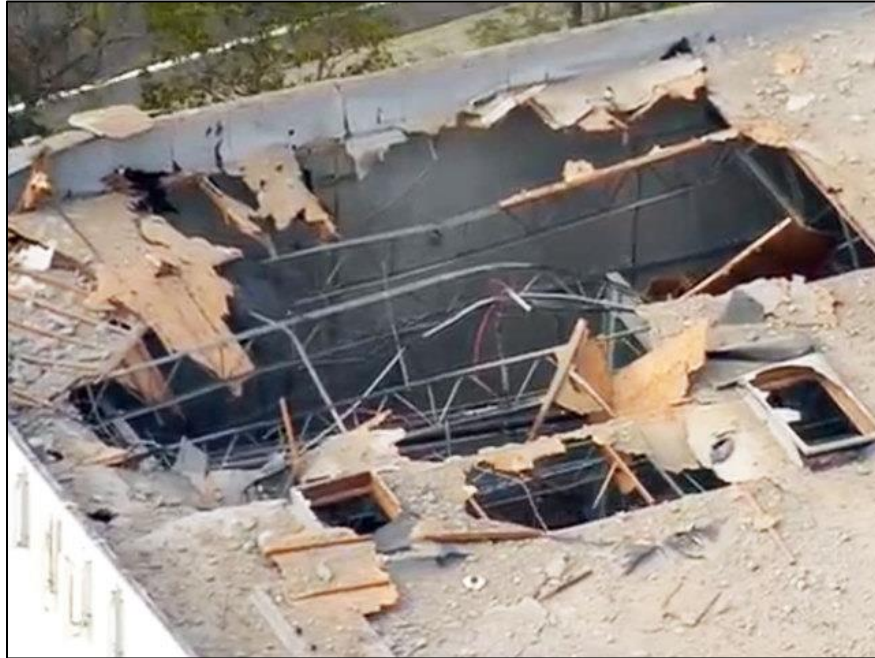
Figure 3: Impression of a FESS damage incident, 10.06.2015, Poway, San Diego, USA - Quantum Energy Storage Corporation [3]
