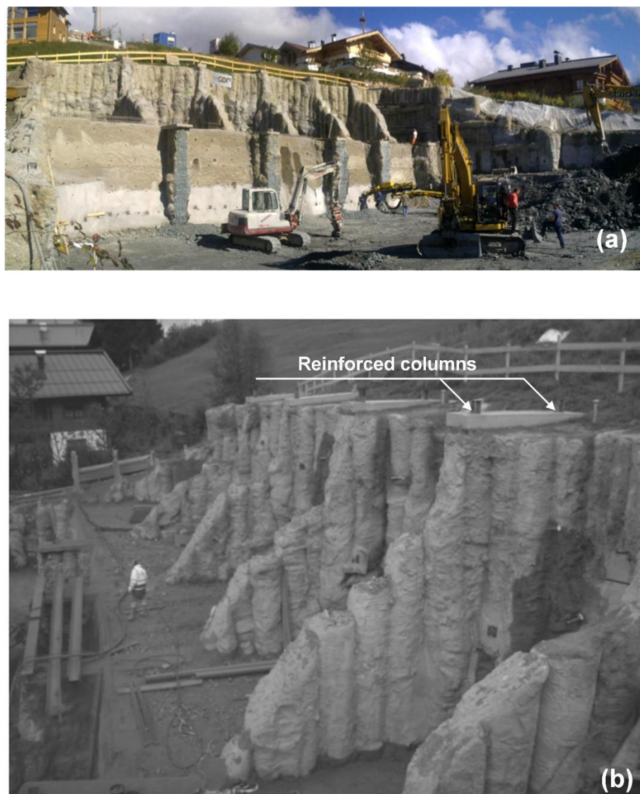
Fig. 50: Structural support system of case history (after Marte et al. 2017)
