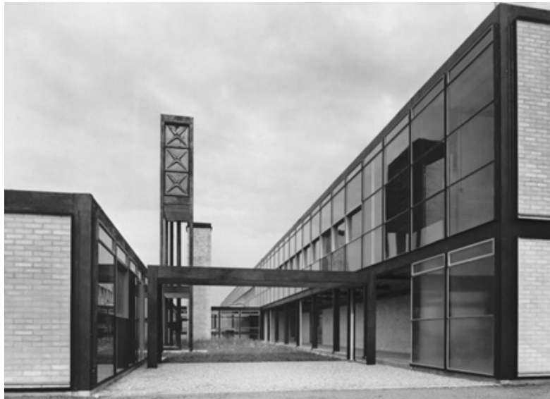
Fig. 6: Hunstanton School by Alison and Peter Smithson is considered to be the first building in New Brutalism expression
