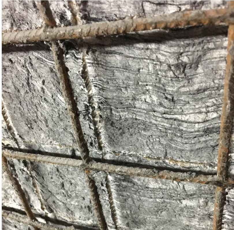
Figure 4.4: Imprint of the reinforcement mesh in the rock mass
