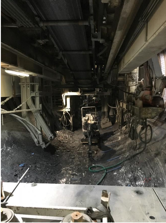
Workspace beneath the TBM
