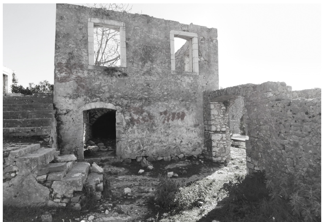
Fig.7: Entrance of the building complex
