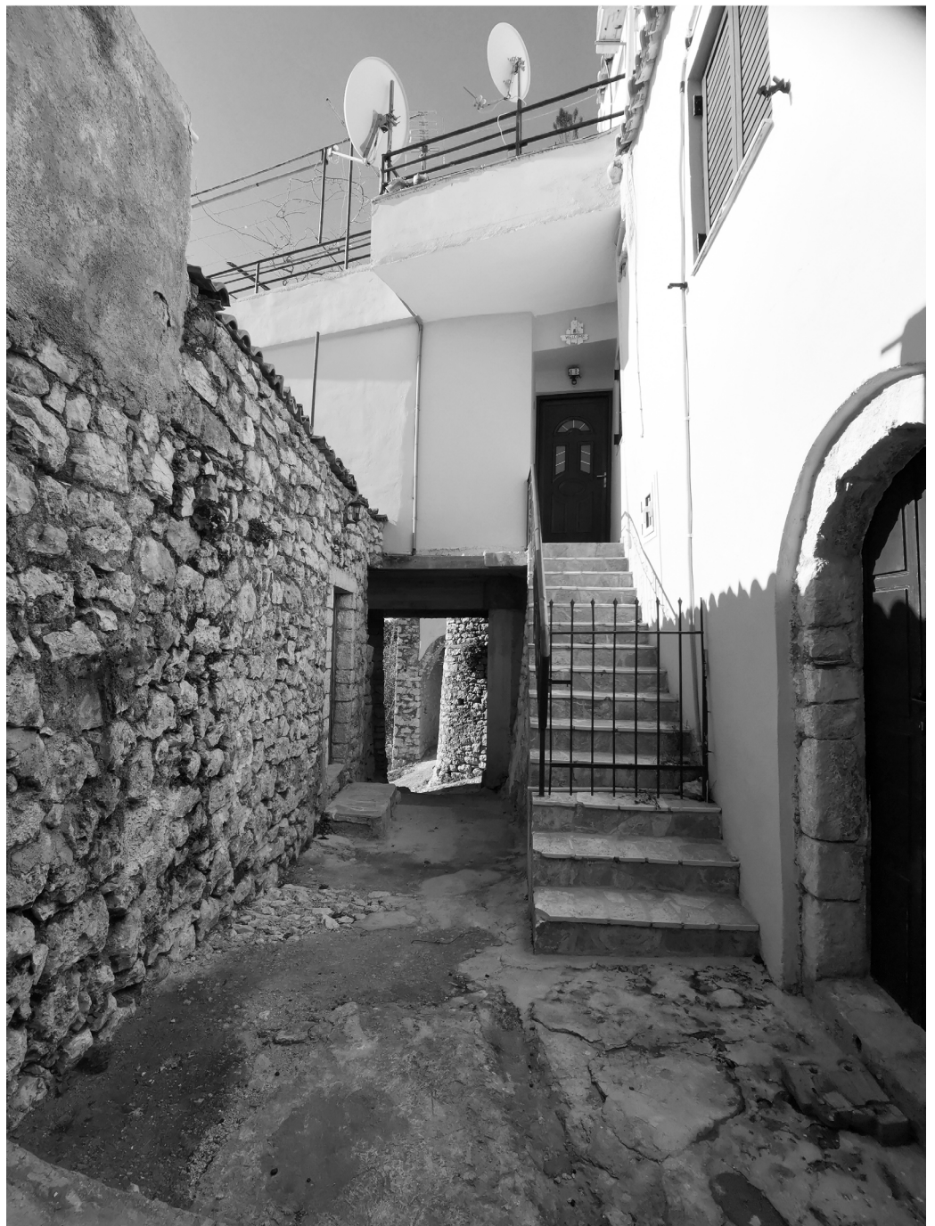
Fig.40: Detail of the interventions on the traditional architecture in the old castle Photo by the author
