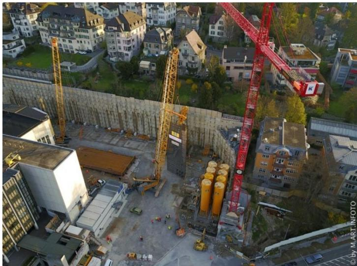
Fig. 28: Deep excavation for GLC building at ETH Zurich 2 (Hechendorfer and Haag, 2018)
