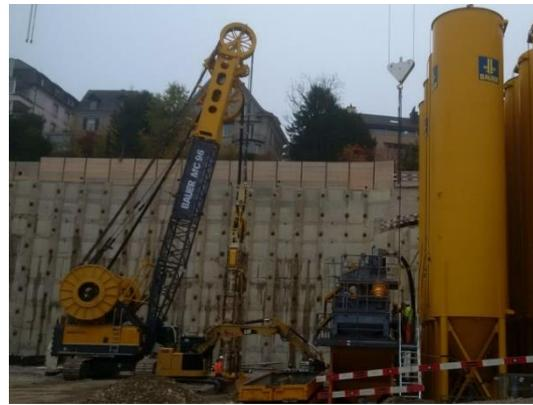
Fig. 2: Anchored building pit with heavy construction machinery (Hechendorfer and Haag, 2018)
