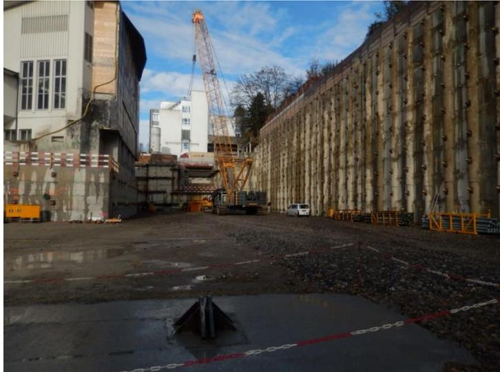
Fig. 27: Deep excavation for GLC building at ETH Zurich 1 (Hechendorfer and Haag, 2018)
