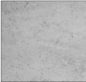
POLISHED CONCRETE used for flooring in the new addition
