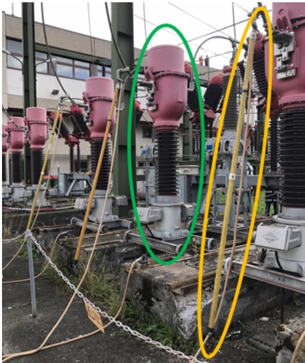
Figure 4.3.: Minimum Oil Circuit Breakers - Combined Transformers (green) and the Earthing Set (yellow)
