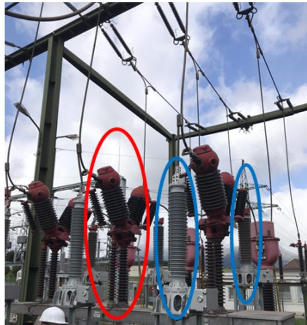
Figure 4.4.: Voltage Measurement Before and After the Circuit Breaker (red) via Ohmic-Capacitive Voltage Dividers (blue)
