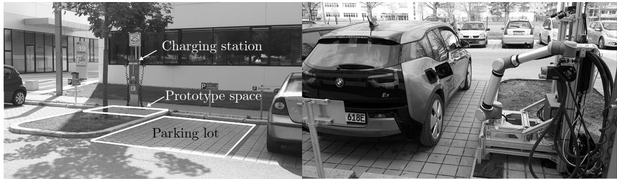
Figure 4.12.: Left: EV charging station at campus of Graz University of Technology. Right: Charging station outdoor test setup.
