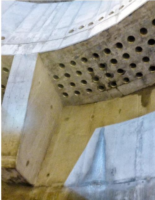
Figure 6-97: Waterfall-dampening device, prototype of surge tank Krespa (courtesy of Illwerke AG)
