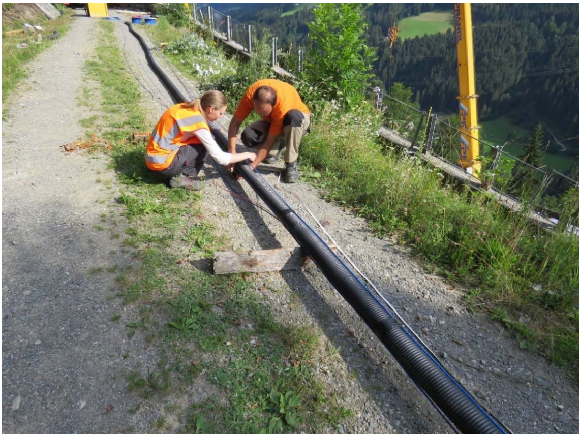
Fig. 76: Installation of the fibres along the corrugated pipe
