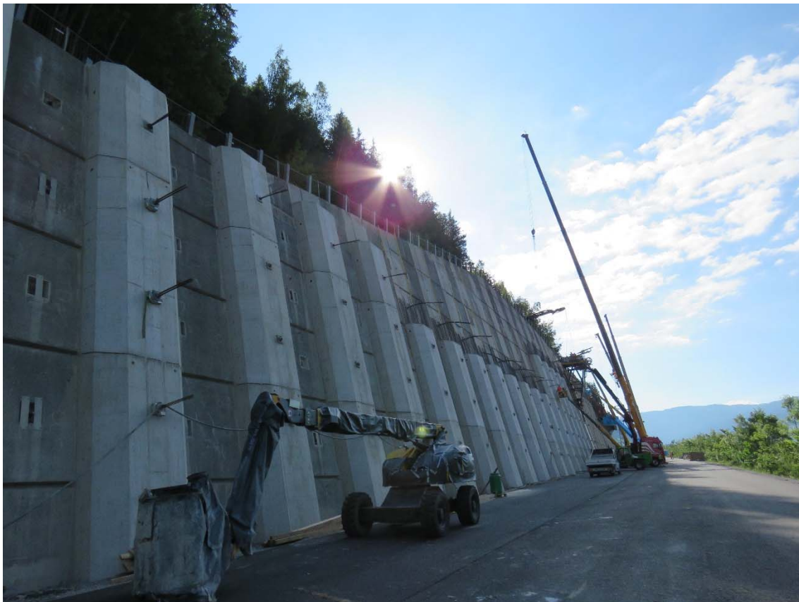
Fig. 74: Retaining wall where the monitored anchor was installed
