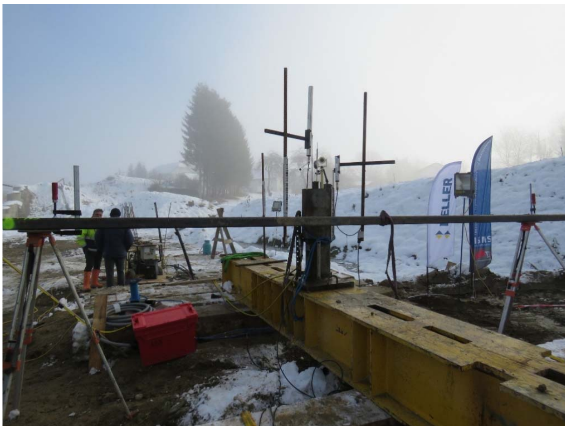
Fig. 31: Pullout test of anchor 1A
