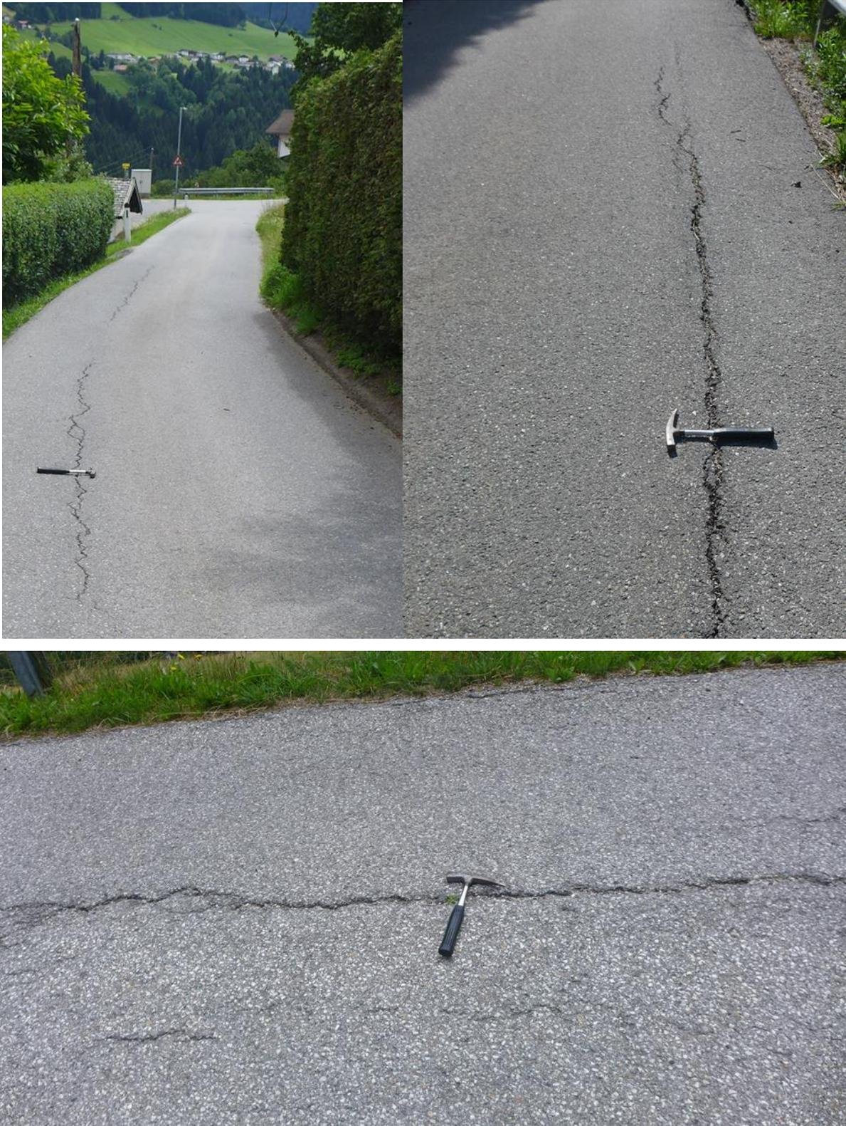
Figure 30: Several examples for cracks in the roads; Outcrop 123 ( Left) and Outcrop 132 (Right) are located in Tauogert, Sellrain; Outcrop 155 (Below) is located in Durögg, Sellrain (outcrops referenced in the large map at the end of the thesis)
