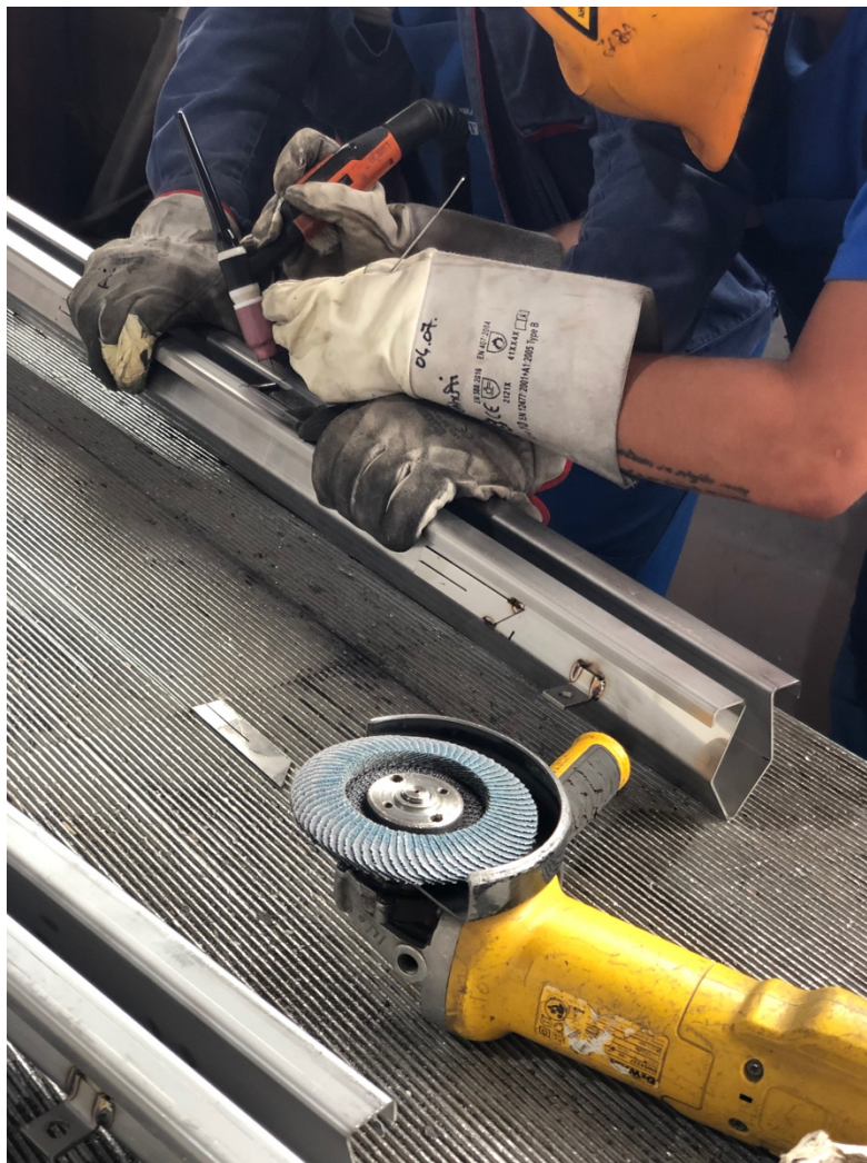
Figure 89 - SRSA welding (Source: Own picture)
