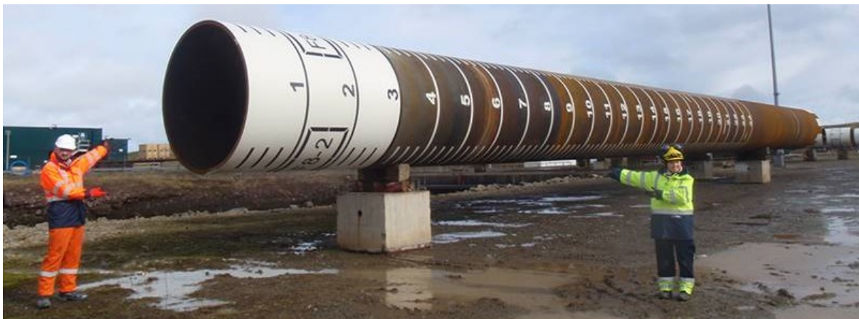
Figure 2.3 Large diameter open-ended steel pile. Source: (BOWL 2011)
