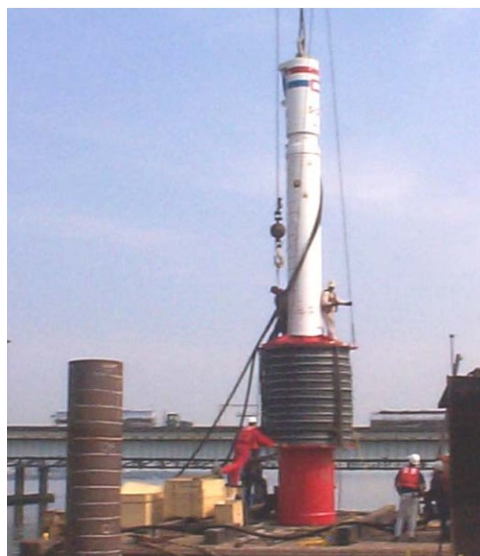
Figure 2.21 Noise shroud for IHC hydrohammer. Source: (Hannigan et al. 2006)
