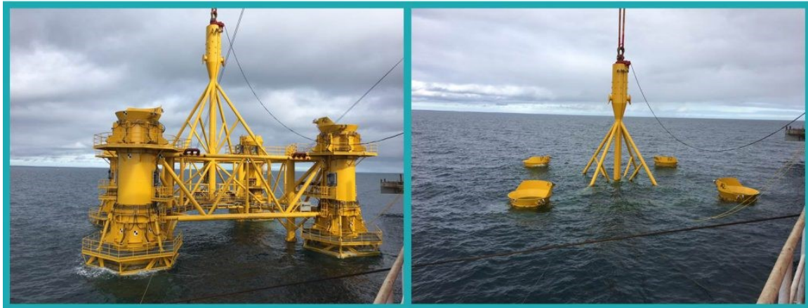
Figure 4.4 Pile Installation Frame (PIF). Source: (BOWL 2017)
