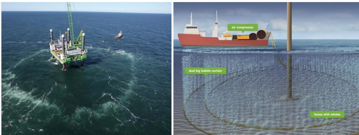
Figure 2.23 Bubble curtains used for noise mitigation. Source: (Rumes et al. 2016)
