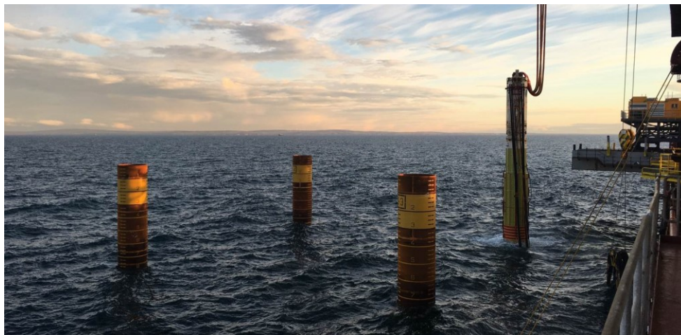
Figure 4.6 Stabbed piles ready for hammering. Source: (Journal John O’Groat 2017)
