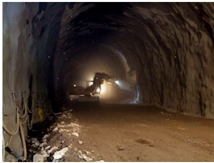
Figure 3.3: Road conditions in Gleinalmtunnel.
