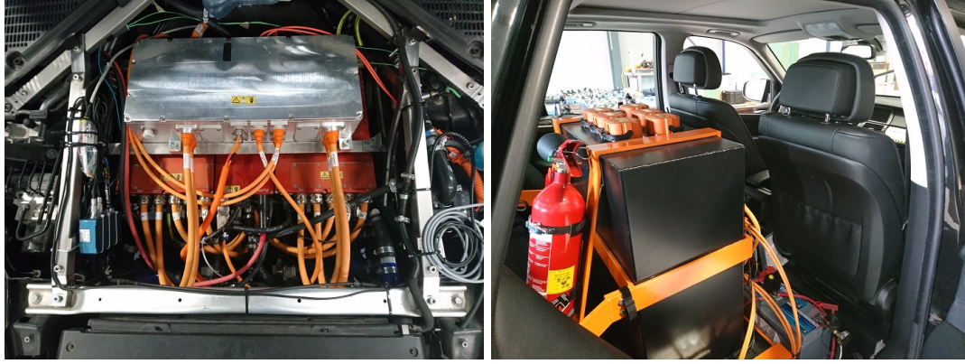
(a) Engine compartment of the refitted BMW with all the power electronic devices. (b) Interior of the car with one of the installed battery packs.
