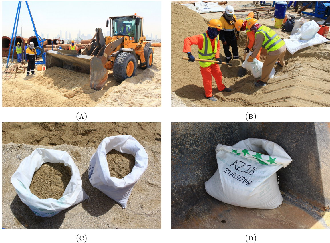
FIGURE 6.5: Excavation of the ditch (A) and taking of the samples (B) in box AZ28 and the bagged and labeled samples from box AZ28 ((C) and (D))
