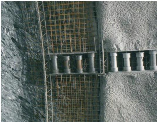
Figure 8: LSC – DSI Underground [9]
