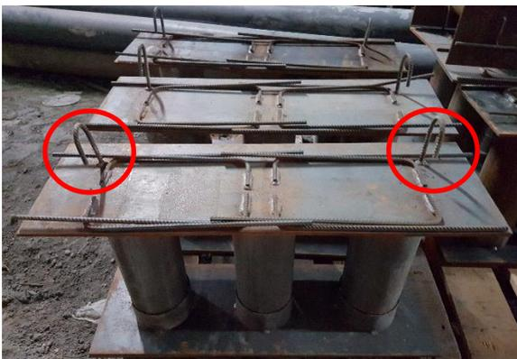
Figure 25: Installation hooks
