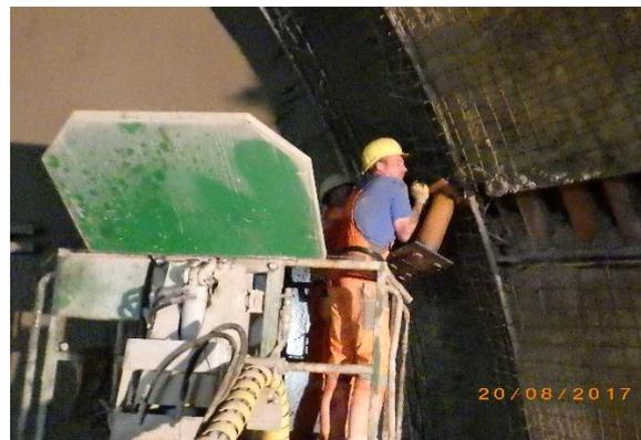
Figure 26: Mounting the yielding element
