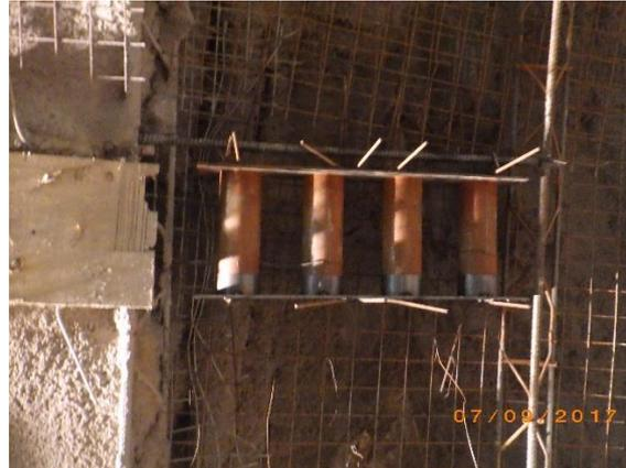
Figure 28: Connection with the first layer of wire mesh
