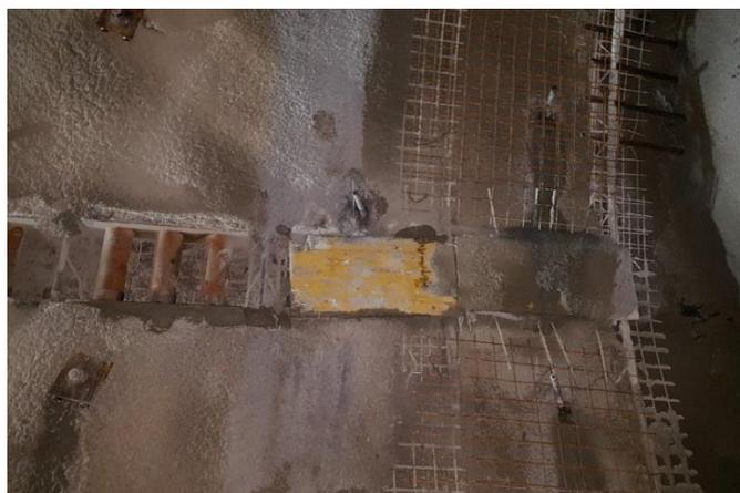
Figure 31: Connection with the second layer of wire mesh
