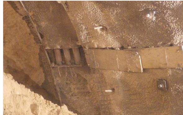
Figure 30: Applying the shotcrete
