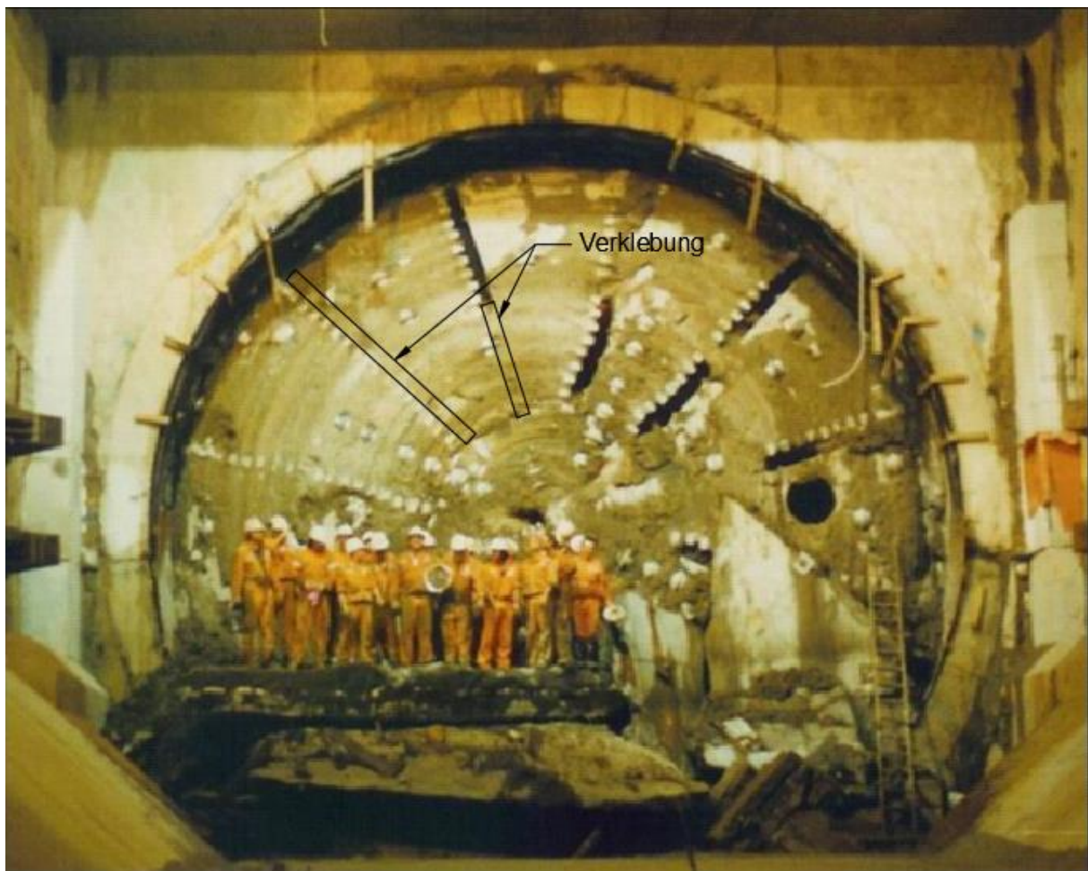
Abb. 1: Verklebtes Schneidrad, Sydney Airport Line - Slurry TBM 10.8 m Diameter, break-out (nach Azzam et al., 2012)
