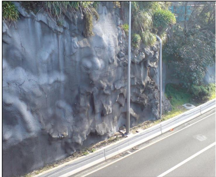
Figure 1: Shotcrete-stabilized cliff wall (Tikkanen et al., 2019)
