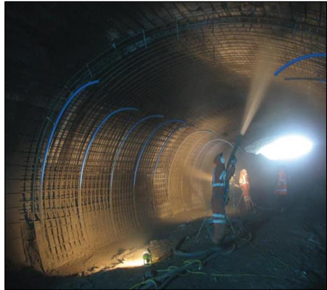
Figure 2: Primary tunnel linings (Sprayed Concrete Association, 2016)
