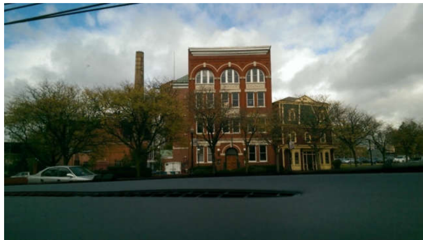
Figure 33, Matt Brewery, which utilizes GE for cooling one of its warehouses. The reason for using GE was innovative nature of the enterprise, as well as an accident which required refurbishment. The company decided to use RES for this purpose, according to the interviewee [42] 118 , source: A. Jovanović
