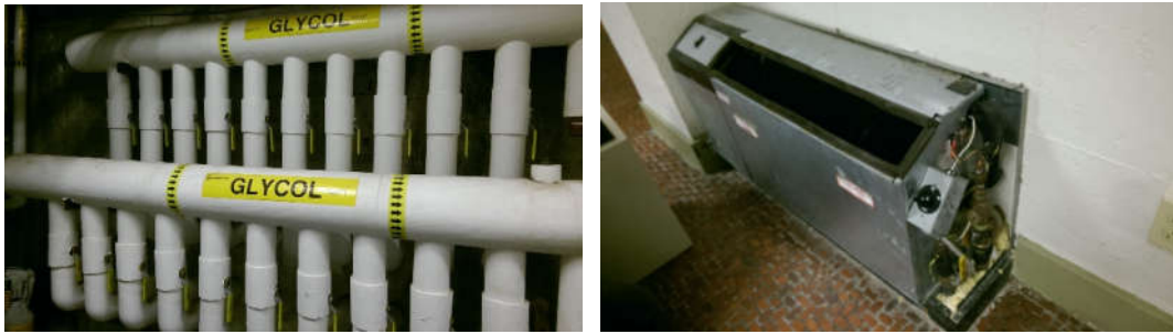
Figure 31c and 31d, photos of the geothermal system (pipes with the fluid and radiators in the hallway)
