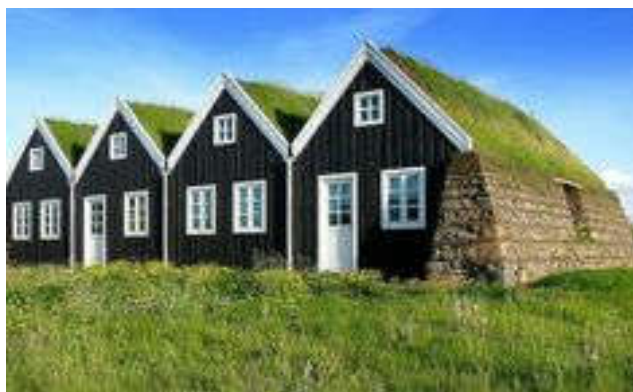
Figure 88, Old turf house principles (burstabær), attached to each other to save energy, keep warm and lower the surfaces exposed to wind and cold
