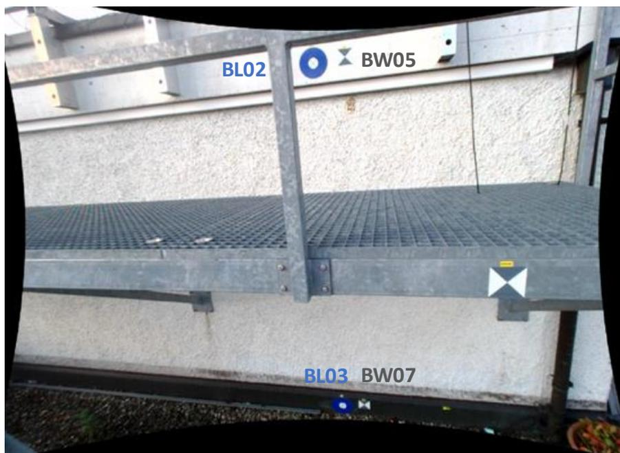
Figure 68: Two different types of targets, BL02 and BW05, BL03 and BW07
