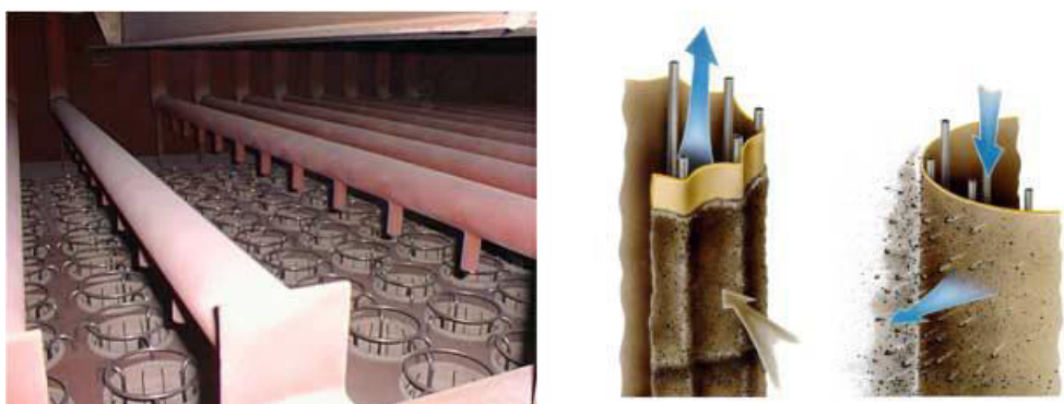
Figure 17: Installed bag house filter (left) and working principle (right) 52
