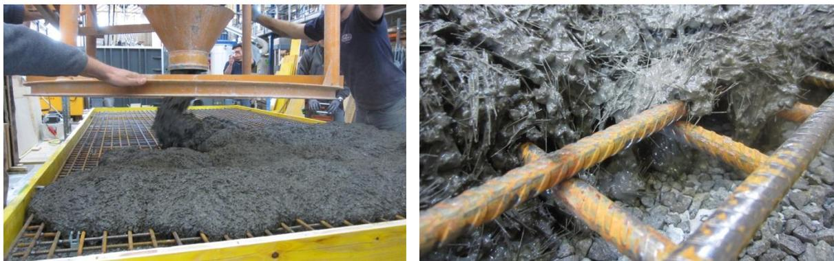
Figure 251: application of the fresh concrete with crane bucket
