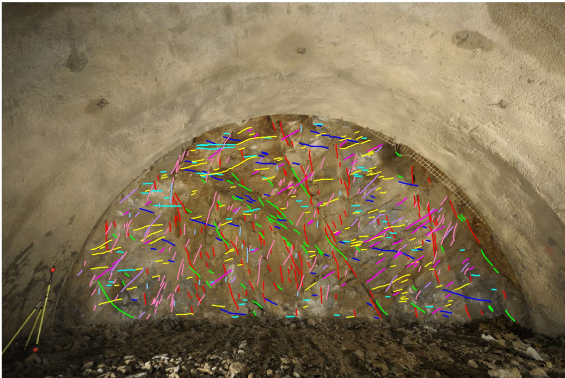
Figure 3.3: Resulting joint trace map from the pixel-based joint trace detection in Case Study I; the lines represent 2D joint traces according to changes in shading and colouring of the input image; the single joint traces are coloured according to the different orientation cluster, in total nine different clusters are distinguished.
