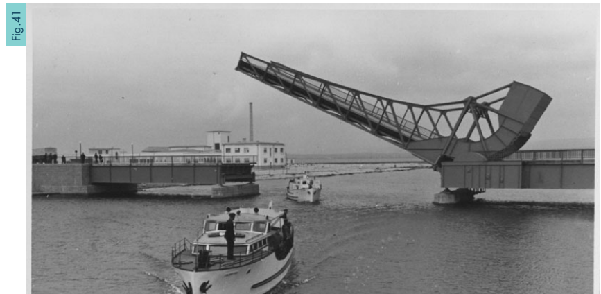
A modern movable iron bridge was constructed. With the help of powerful electric motors, it opened in just two and a half minutes, with an opening width of up to 30 m. 4
