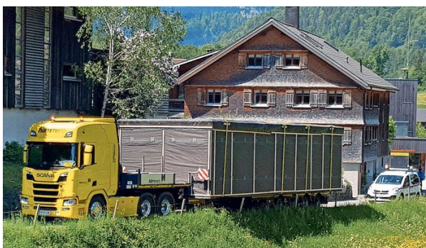
Abbildung 4.8 Transport Raumzellen, [34] [31]
