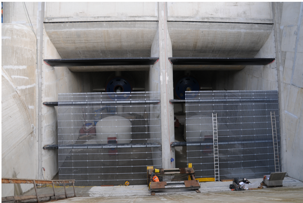
Figure 2.9: Construction of a trashrack structure at a ROR (Source: Institute of Hydraulic Engineering and Water Resources Management, TU Graz).
