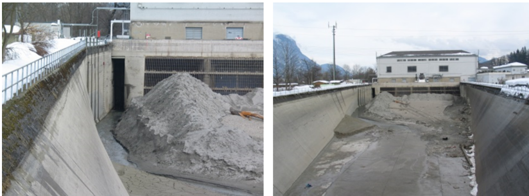
Figure 2.13: Sedimentation in front of the intakes (Source: TIWAG).
