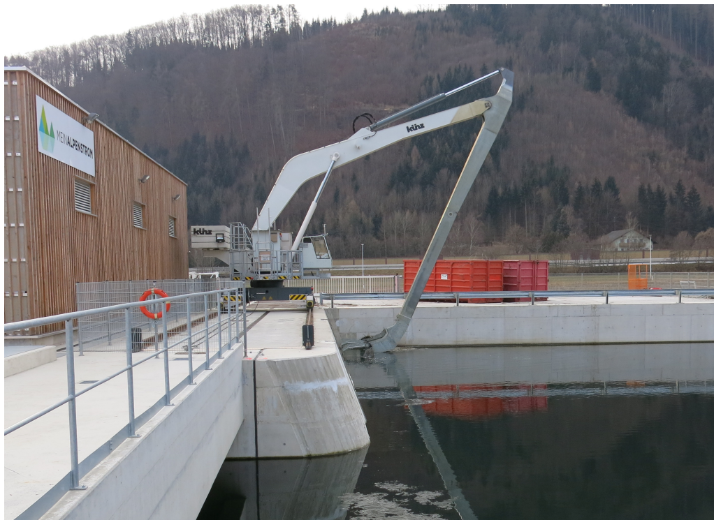
Figure 2.10: Trashraking system using hydraulically articulating arm at a ROR (Source: Institute of Hydraulic Engineering and Water Resources Management, TU Graz).
