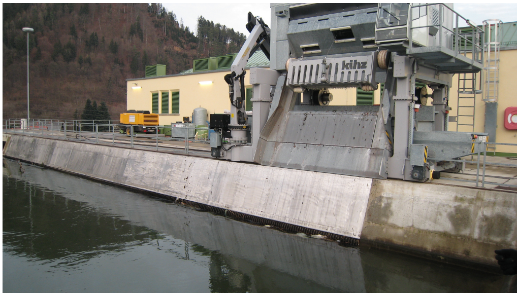
Figure 2.11: Alternative trashraking system at ROR (Source: Institute of Hydraulic Engineering and Water Resources Management, TU Graz).
