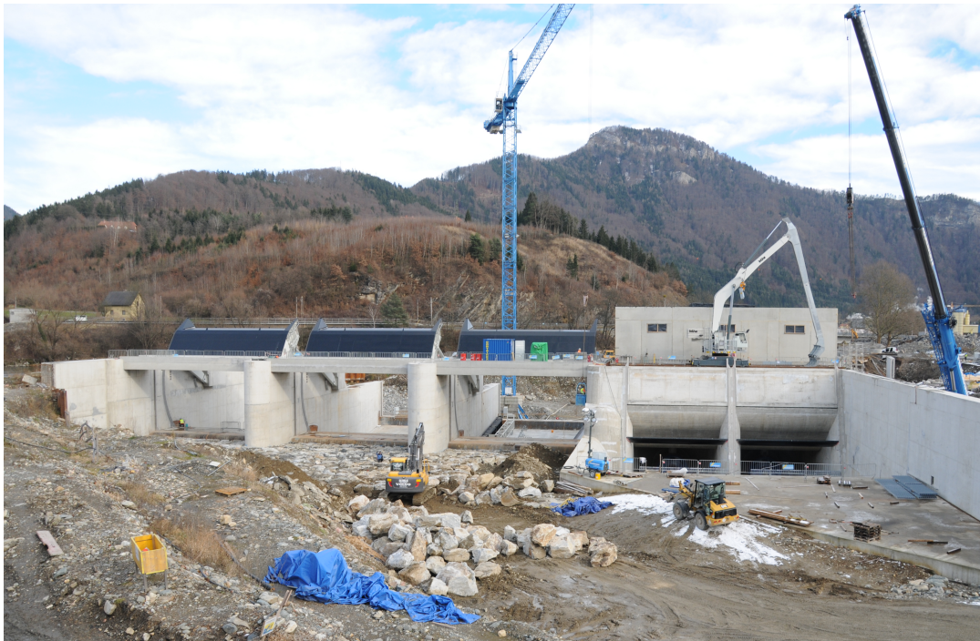
Figure 2.2: A ROR with forebay under-construction (Source: Institute of Hydraulic Engineering and Water Resources Management, TU Graz).
