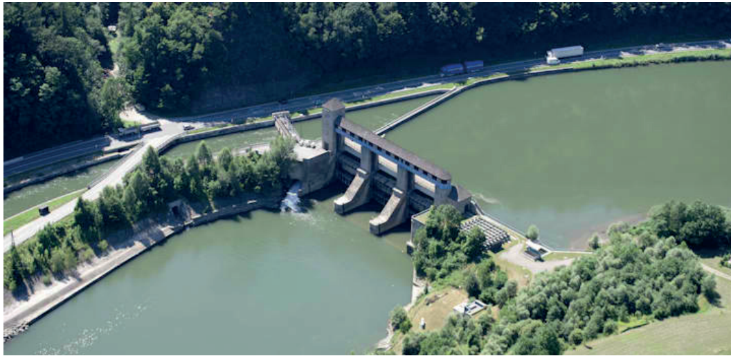
Figure 7.2: Weir and diversion channel of the Zlatten reservoir in Styria, Austria
