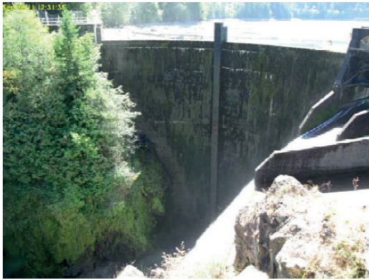
Figure 4.11: Glines Canyon Dam before deconstruction in September 2011 (USSD, 2012)
