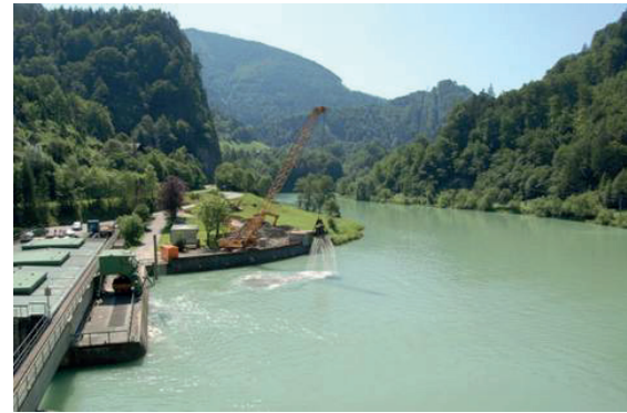
Figure 8.4: Dredging at the turbine inlets in July 2009
