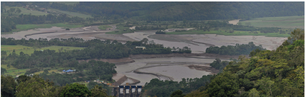
Figure 7.5: Angostura reservoir in Costa Rica with lowered operation level at a flushing event
