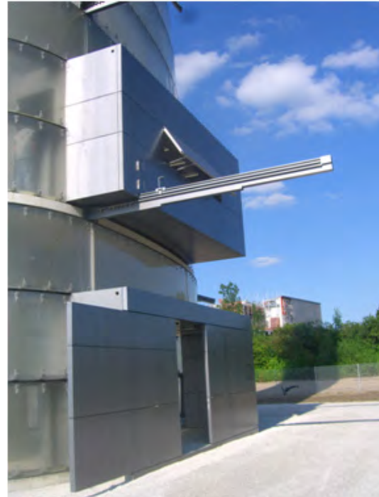
Figure 6: entrance and box
