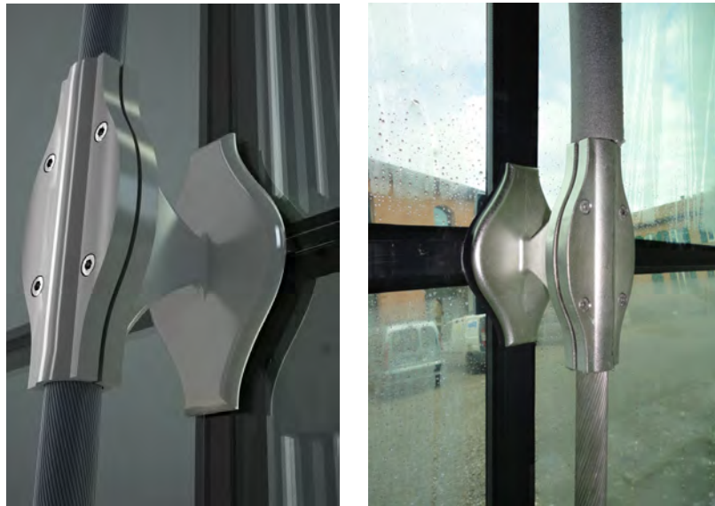
Figure 4: Glass fixing and cable clamp. Rendering (left); Assembled cast piece (right) - (Werner Sobek Stuttgart)
