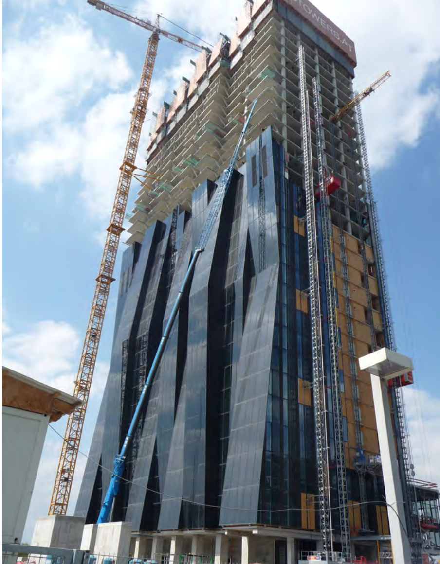
Figure 10: Façade DC – Tower 1, Status of construction end of April 2012
