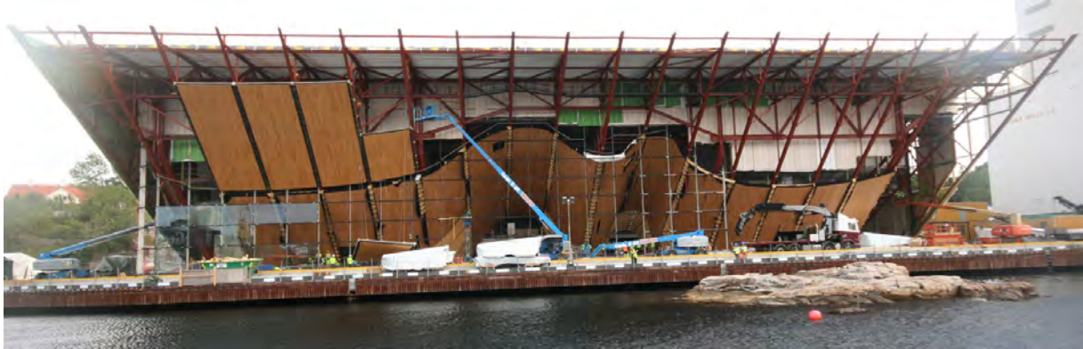
Figure 3: The façade during erection ( Trebyggeriet )
