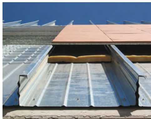
Figures 4 and 5: Steel folded plate as inner skin.
