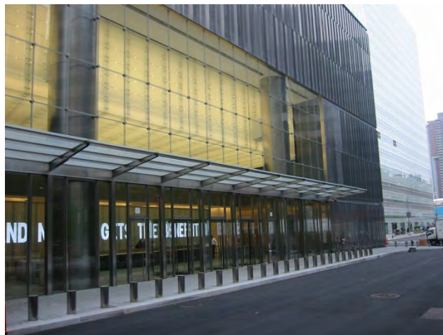
Figure 8: Explosion resistant entrance facade of World Trade Center Tower 7, New York (Gartner)
