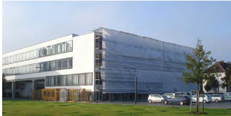
Figure 4: Bauhaus-building during renovation.
