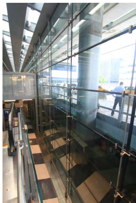
Figure 6: Clamped connection, Chicago Airport (Gartner)
