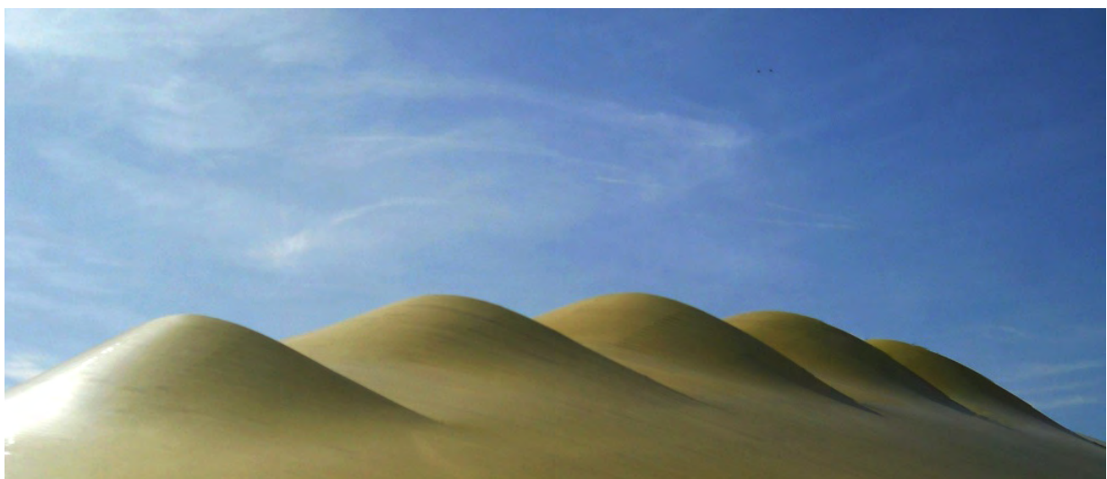
Figure 5: View of the aluminium roof (Teleya)
