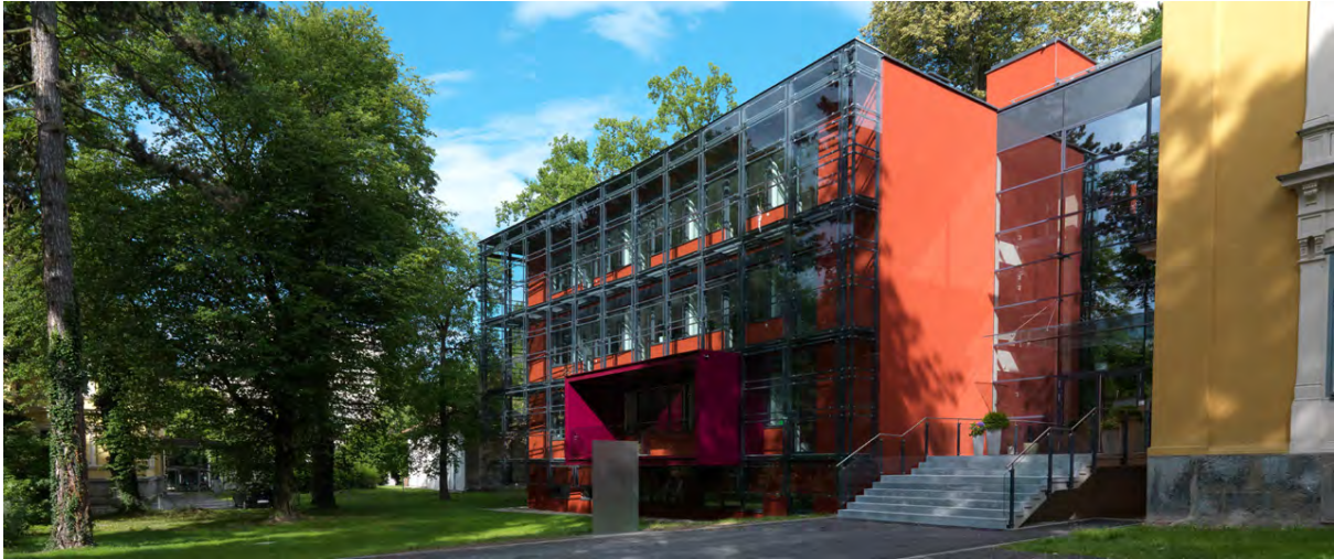
Figure 6: Hartenaugasse office building, façade. Photo Gerald Liebming
