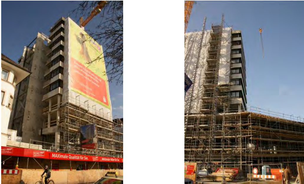
Figure 1 a & b: Dismantling of the Concrete Façade Elements
