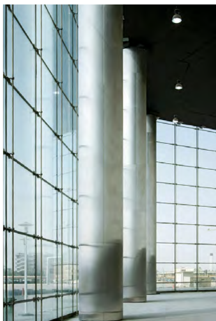
Figure 3: Cable net facade with straight cable direction (type 1): Hamad Medical City, Doha, Qatar (Gartner)
