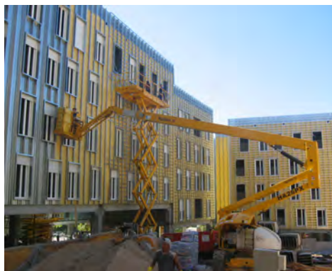
Figures 4 and 5: Steel folded plate as inner skin.
