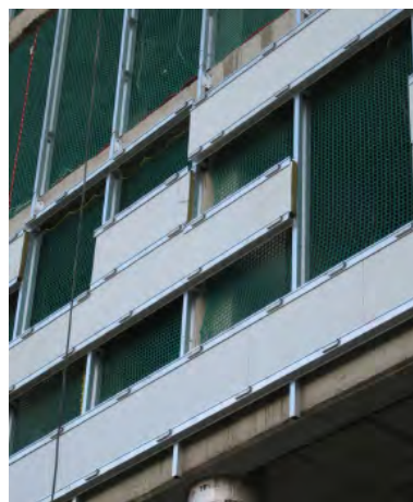
Figure 3: Wind load bearing inner skin.
