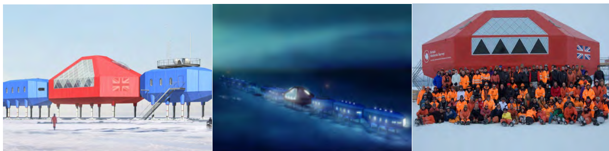
Figure 9: British Antarctic Survey Research Station Halley VI.
