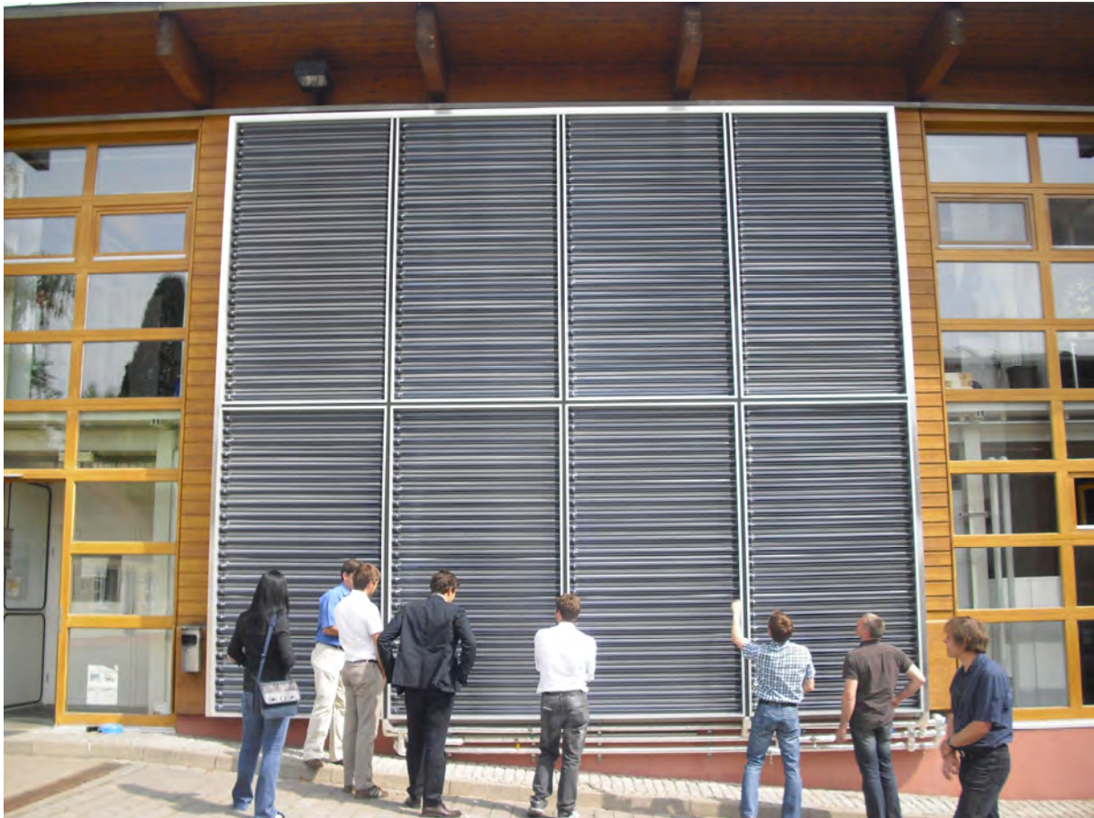
Figure 4: Test facade located in the area of Ritter Solar, Dettenhausen
