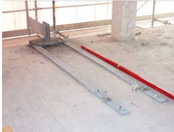
Figure 5: Steel Fins are fixed to the Concrete Floor by Anchors
