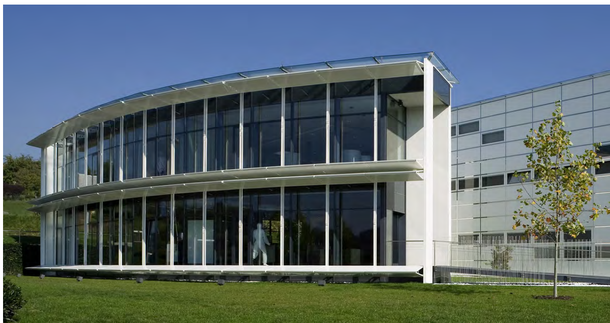
Figure 1: Kiefer Technic façade, completely opened. Photo Paul Ott
