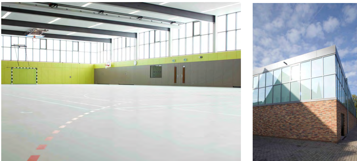
Figure 6: Typical daylighting application at a gym in Herzebrock.
