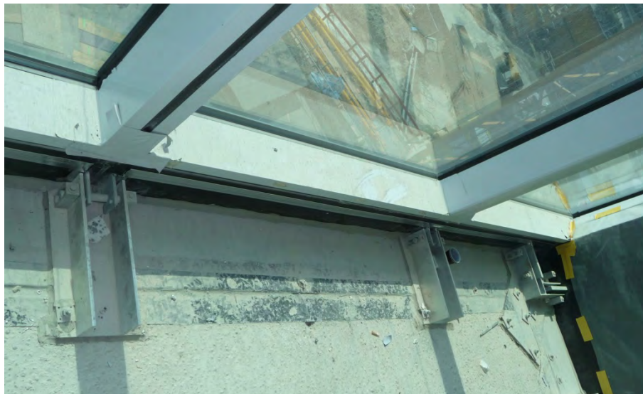
Figure 12: Detailed bracket DC Tower 1
