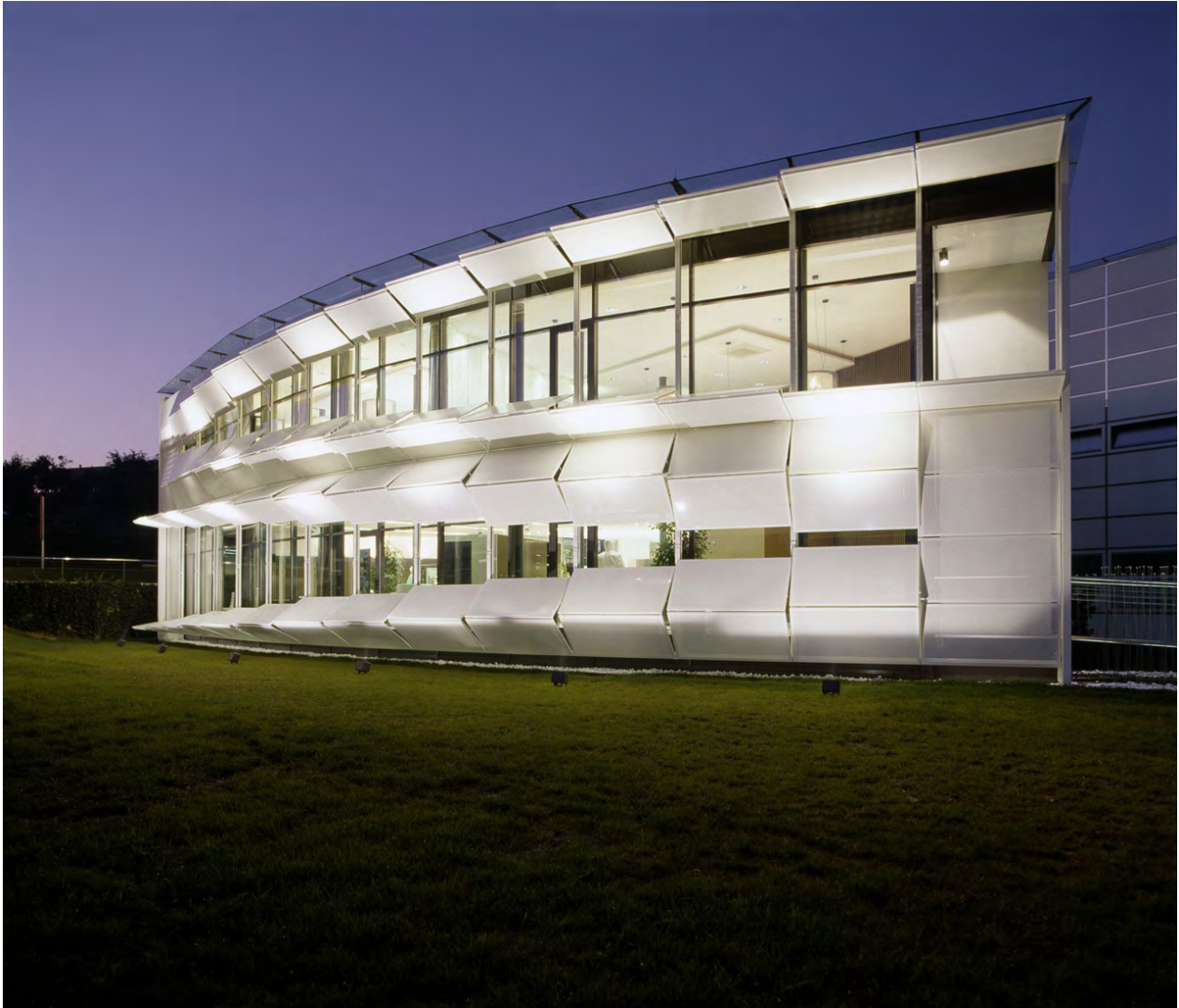
Figure 3: Kiefer Technic façade at night. Photo Paul Ott
