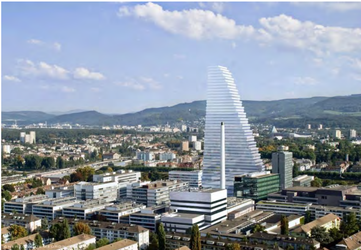
Figure 1: The prospective tallest high-rise in Switzerland with 178 meters in height, overview urban layout, High-rise F. Hoffmann-La Roche
