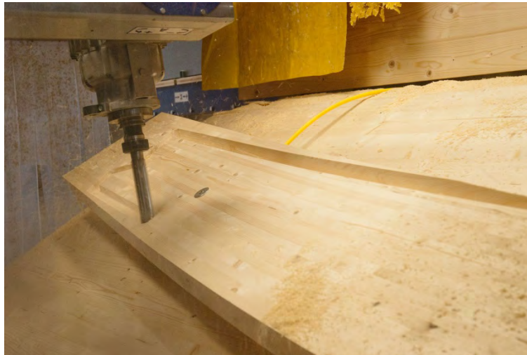
Figure 5: CNC-milling a curved glue-laminated timber beam ( designtoproduction )
