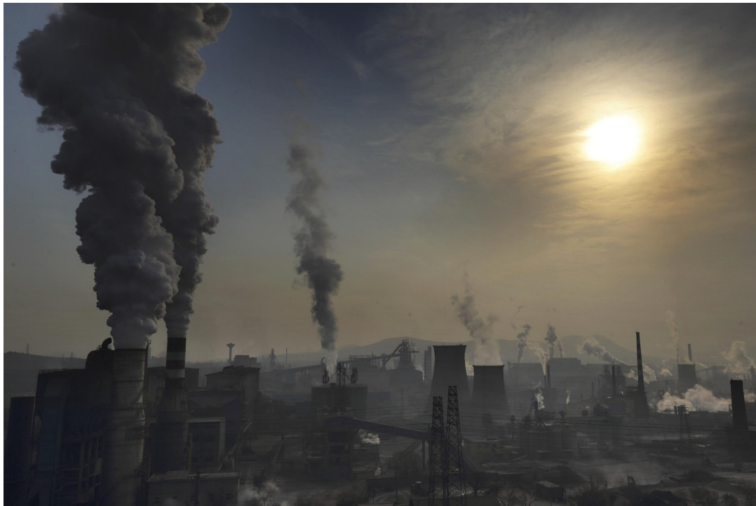
Figure 2.6: Steel plant in Yuanbaoshan, Hebei, copyright by Lu Guang, Greenpeace
