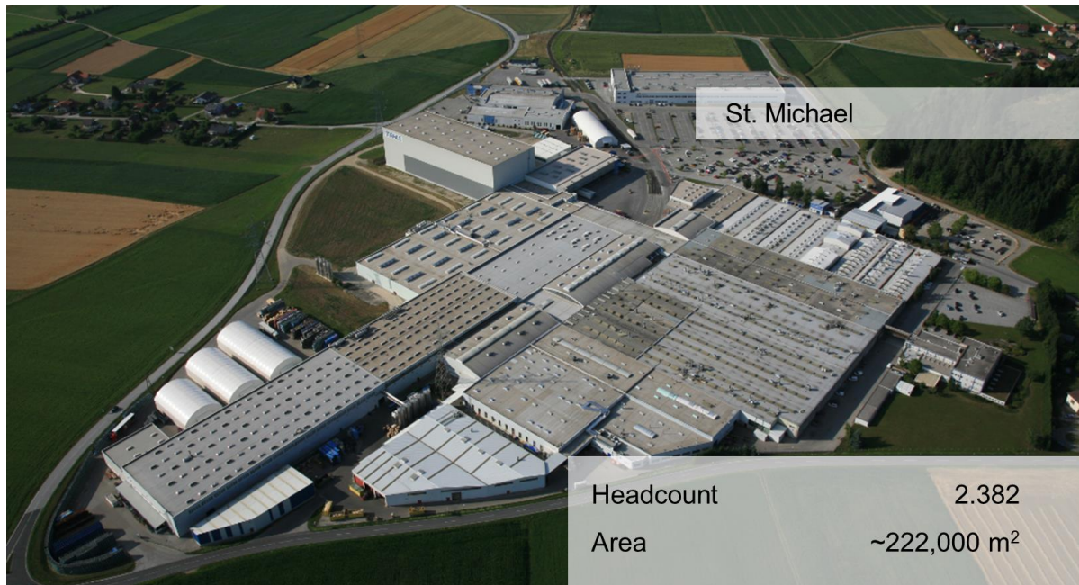
Figure 1-1: Plant of MAHLE Filtersysteme Austria GmbH
