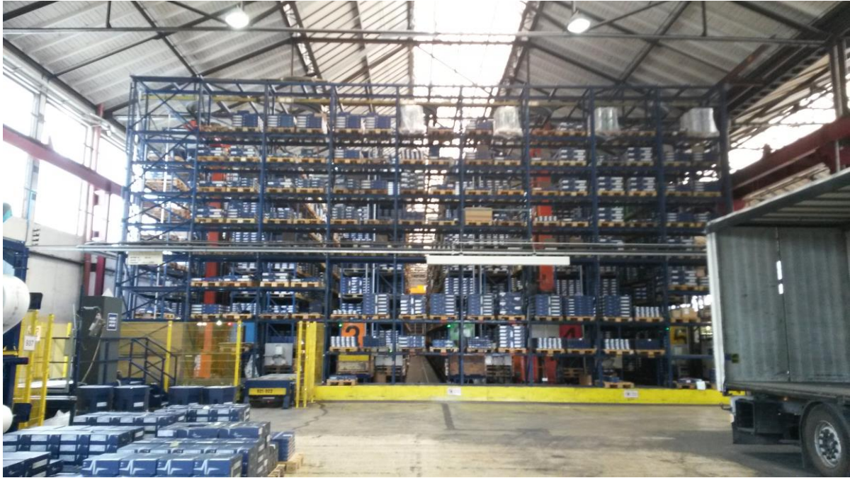
Figure 4-3: High-Rack Storage's front face
