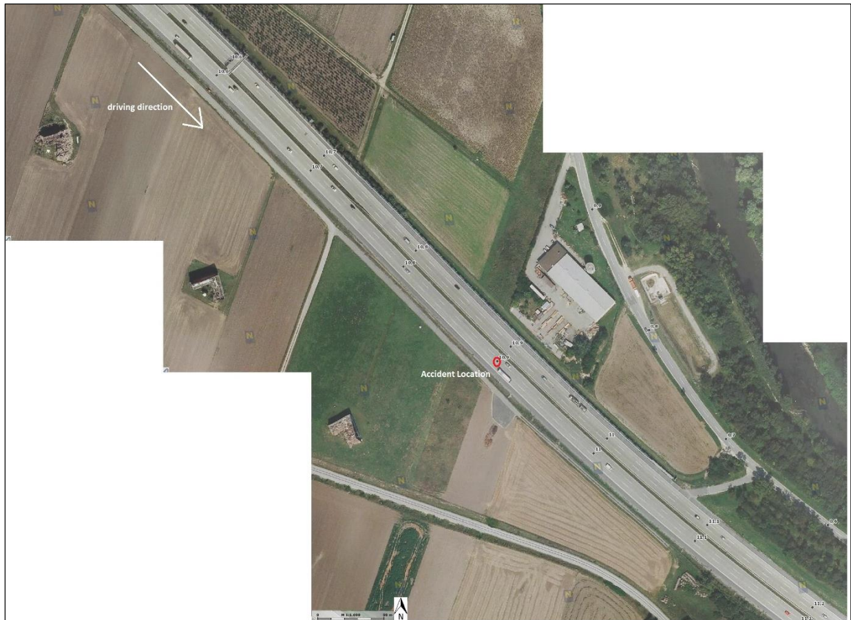
Figure 3-21: Highway section where accident happened [36]
