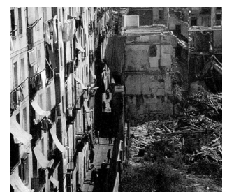
Fig. 24 Rambla del Raval under construction, 1999.
