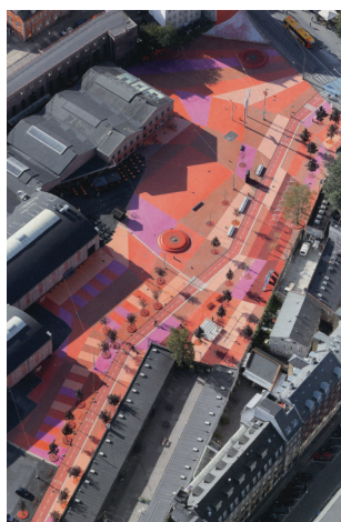
Fig. 5 Superkilen, aerial view. The redesigned public area of the Red Square shows a patchwork of surfaces and a selection of symbolic elements of street furniture.
