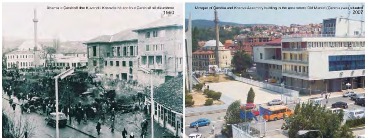
Fig. 35 Two pictures: Demolition of Prishtina bazaar and actual situation - Brotherhood and Unity square (1960)
