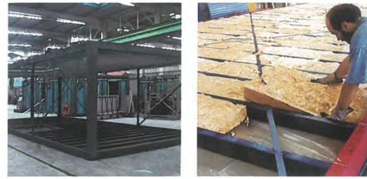
Figure 2-49: Production of steel room modules in a factory. 100
