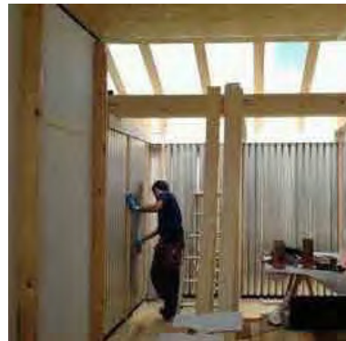
Figure 3-26: Internal alloy tubes in-filled with wet sand in the cavity of the wall. 125
