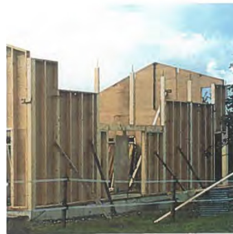
Figure 2-44: Shell, timber frame construction 96
