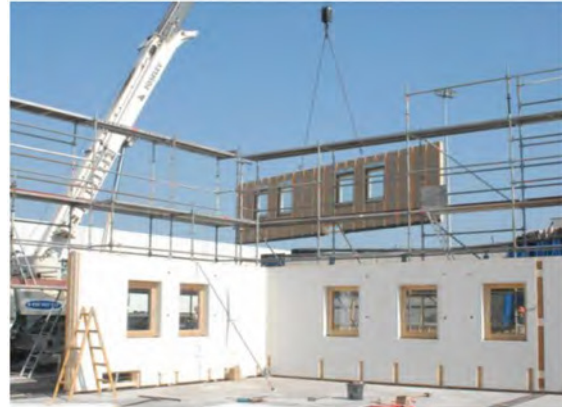
Figure 3-34: Panel construction assembly on site.
