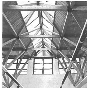
Figure 2-30: Timber space frame roof structure 87
