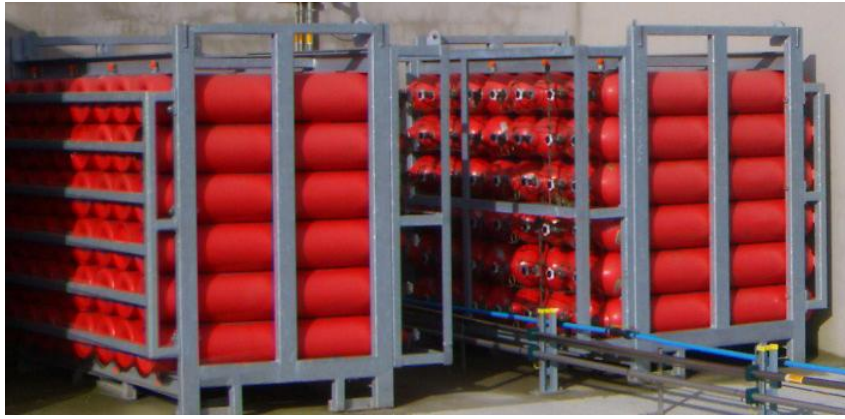
Abbildung 1.3: 200 bar Hydrogen Storage Manifold Cylinder Packs (MCP) [10]
