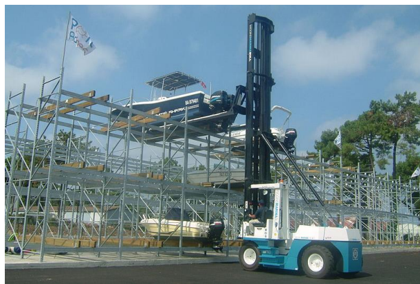
Figure 3-13: Vertical Dry Storage
