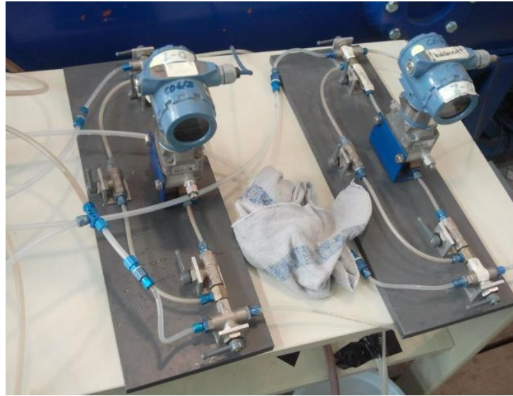
Figure 5.5: Different pressure sensors installed with flushing valves
