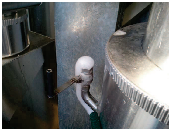
Fig. 4-4: Escape of foam from the absorber (Posch, 2012).
