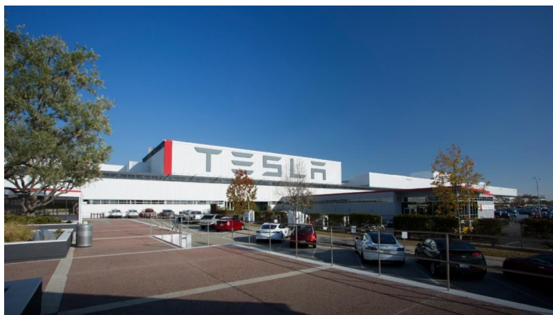
Figure 34 Tesla Motors factory in Fremont, California (The Tesla Motors Team, 2014)
