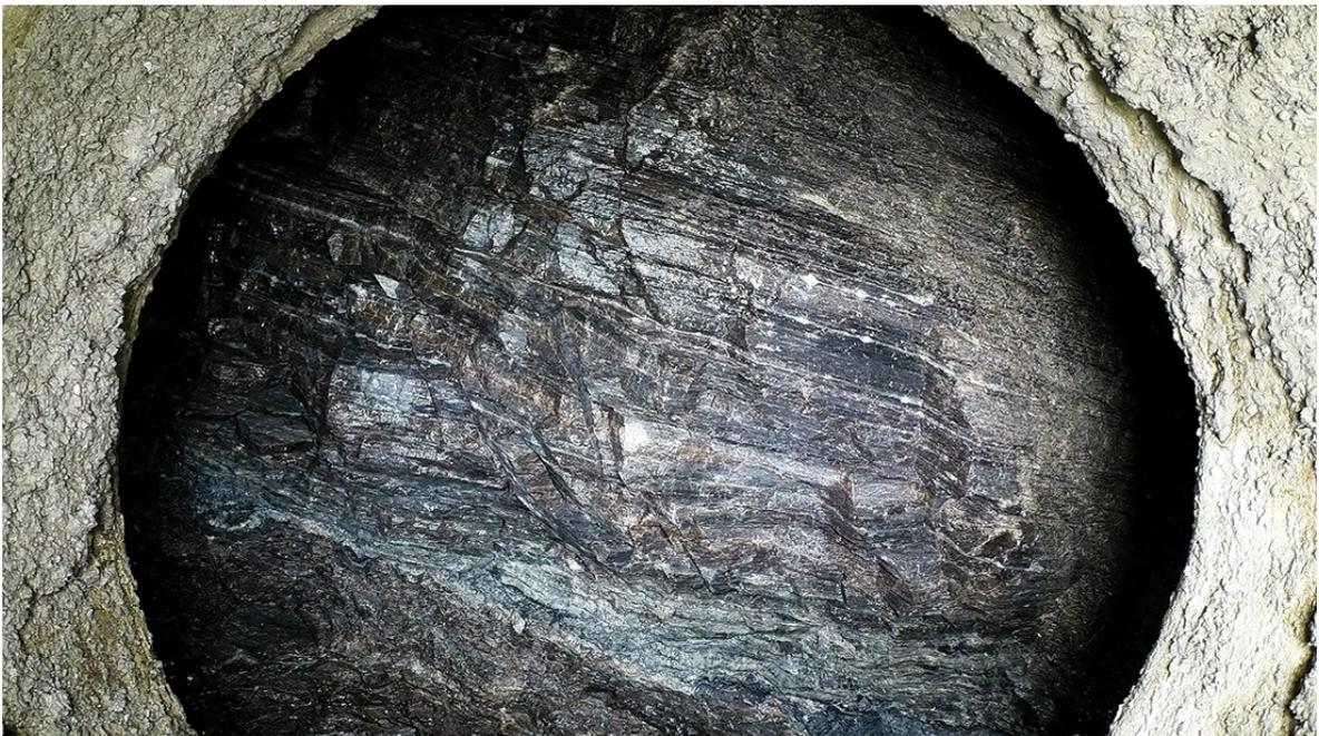
Figure 2.2: Subimage of the video showing a detail of the tunnel face and parts of the inspection opening in the border areas
