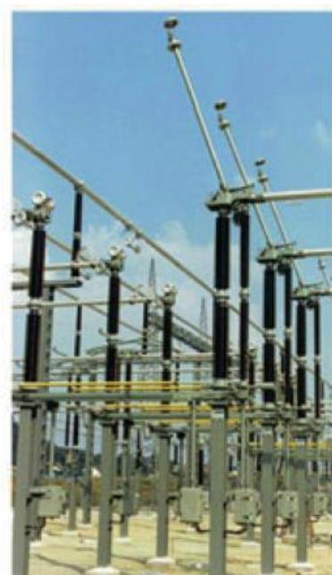
Abbildung 3.6: Pantograph (Scherentrenner - l) [6] – Trenner (r) [9]
