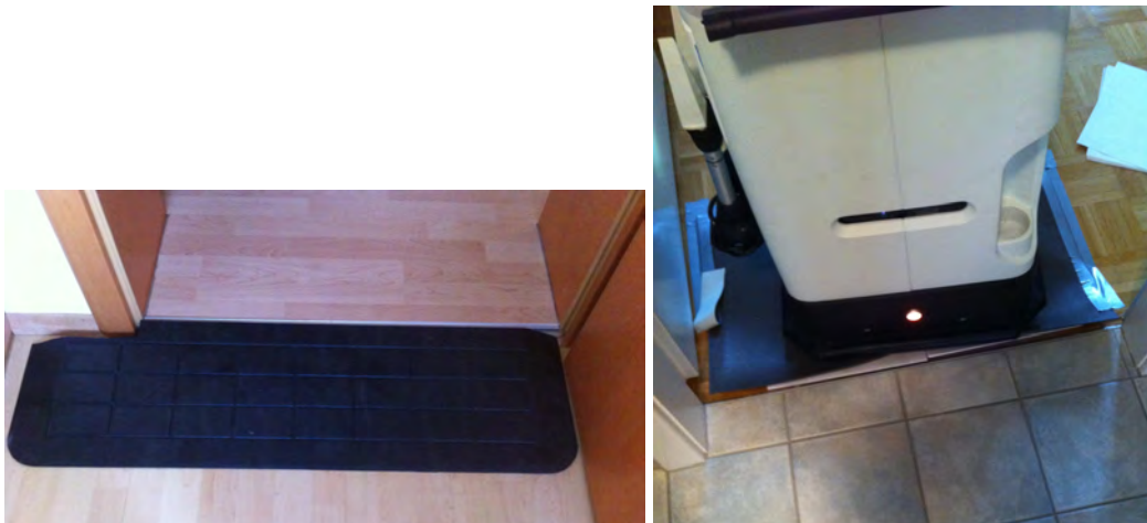
Figure 8. Using ramps to go through thresholds.
