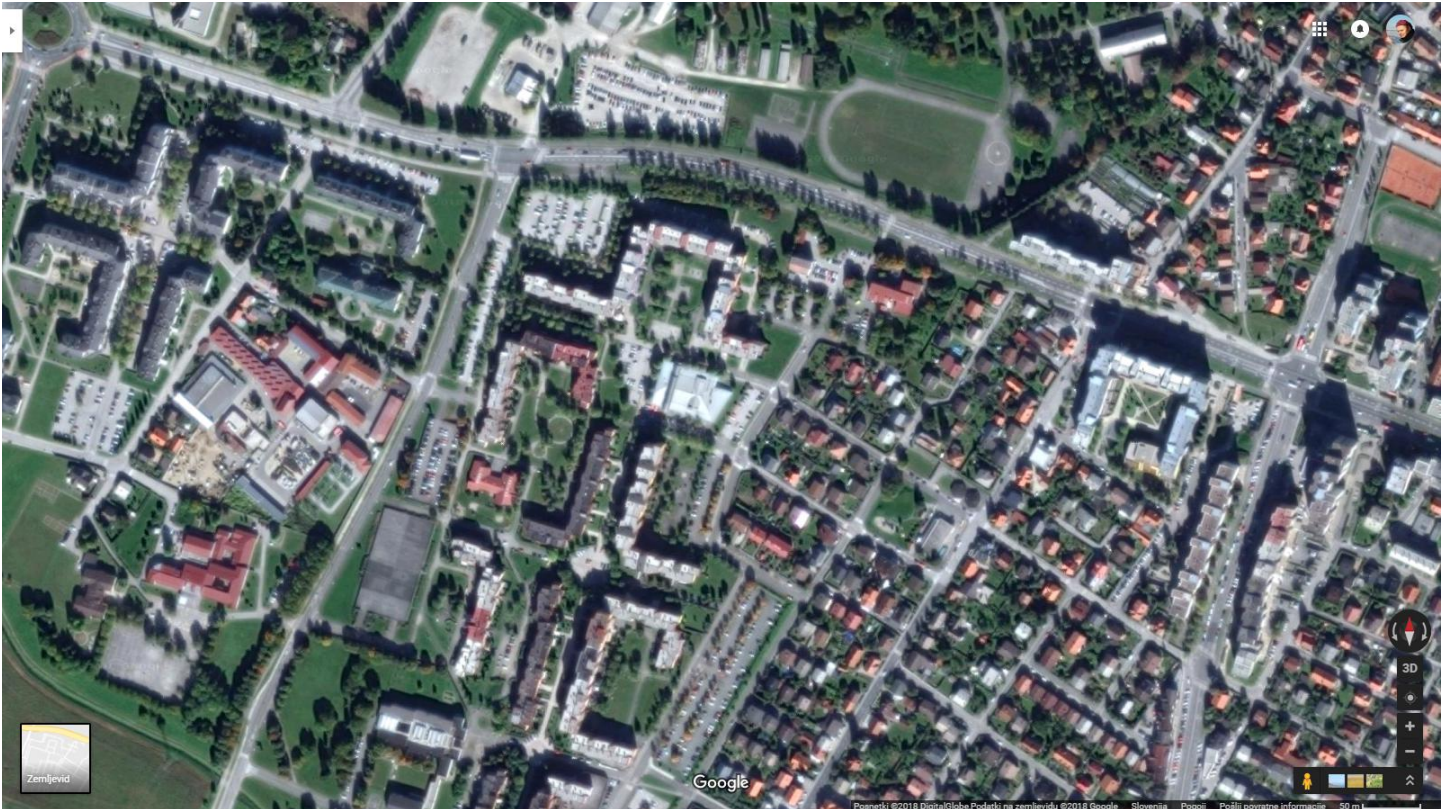
Fig. 6.30 Maribor, Slovenia. The vast Maribor Jug urban development is inserted into irregular tissue. Irregular never became regular with this insertion. Google Maps, ©2018 DigitalGlobe
