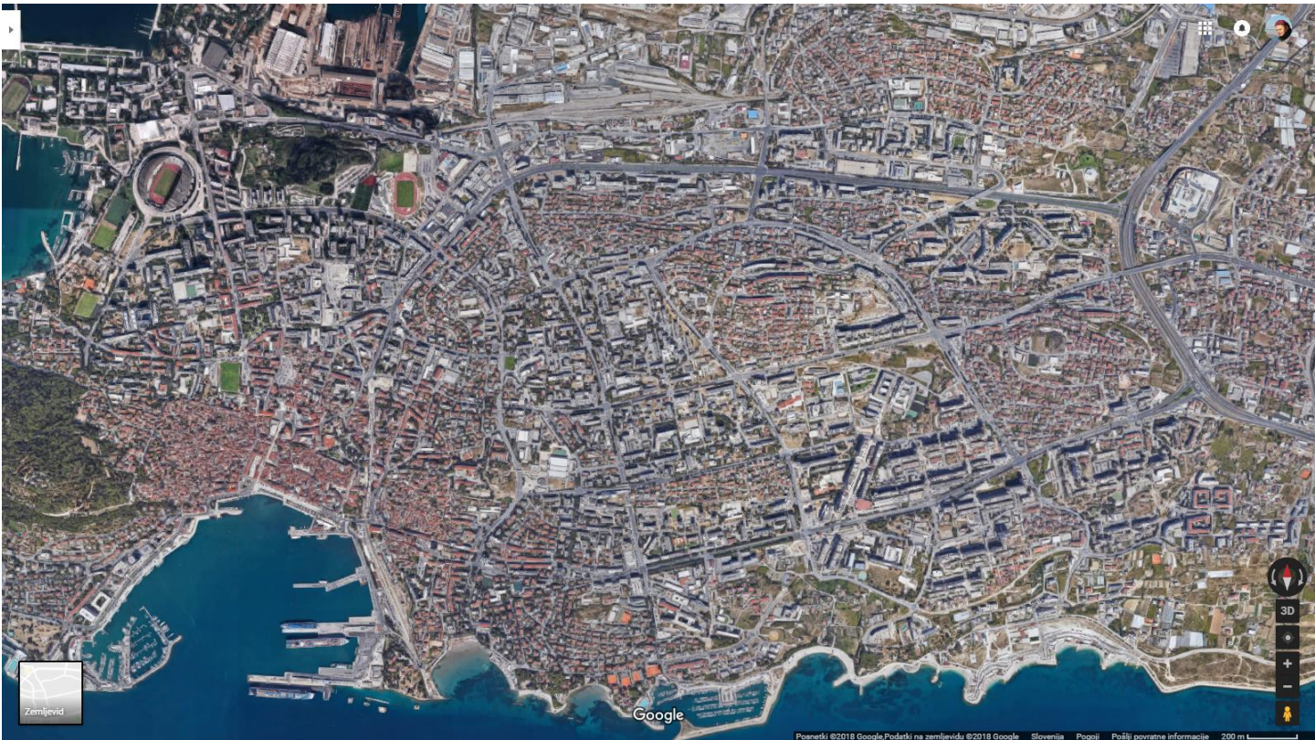
Fig. 6.23 Split, Croatia. The Split II and III socialist extensions completed the city image and structure and considerably improved the inhabitants' spatial standards. Google Maps, ©2018 Google
