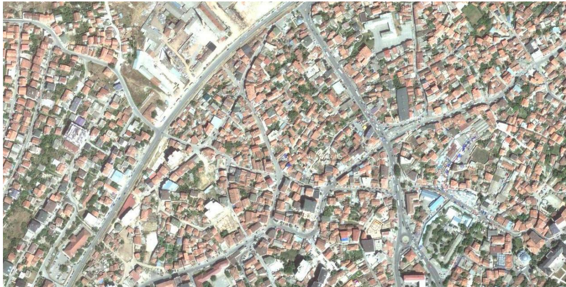
Graphic material 2: the ortophoto of the northern part of Pristina called Tophane reveals a major densification of the structure due to a relatively strong demographic growth (maps.google.com)
