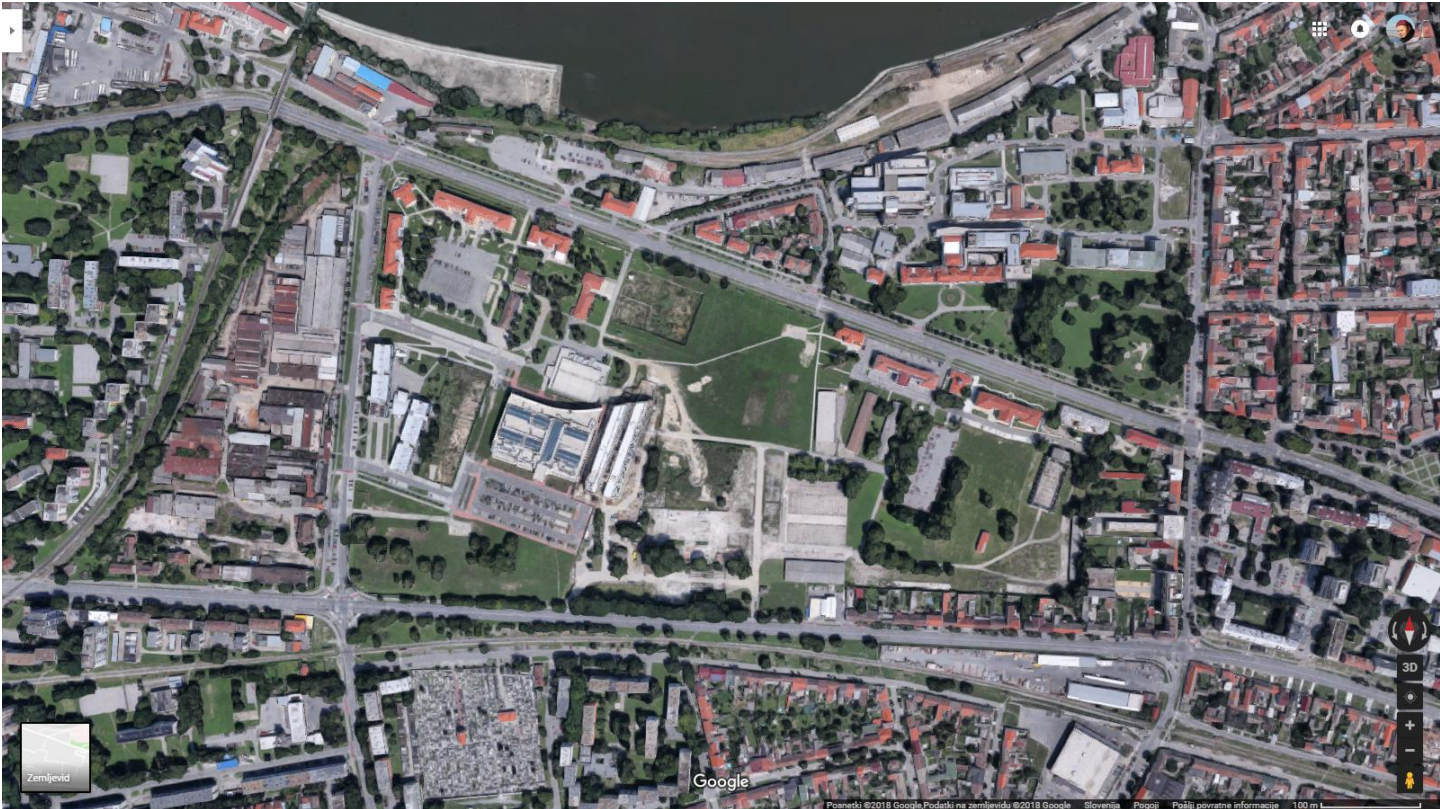
Fig. 6.45 Osijek, Croatia. Former Military barracks, founded in the Gründerzeit period, are being smartly converted to University campus and will eventually form a unity with the neighbouring hospital. Google Maps, ©2018 Google.
